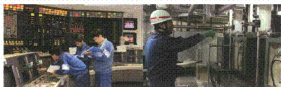
System functional test (inspection of the Unit 7 turbine bypass valve function)
