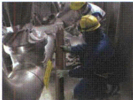
Addition and reinforcement of pipework supports
