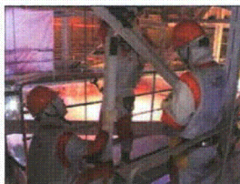
Reinforcement of the truss of a nuclear reactor building roof
