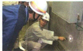
Visual inspection of the wall of the nuclear reactor building
