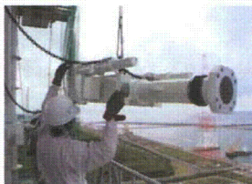
Installation of a vibration control device
